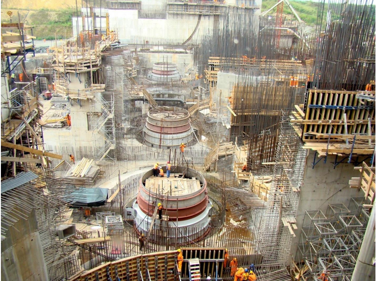
Construction of Bujagali Hydro Power station under PPP project in Uganda
