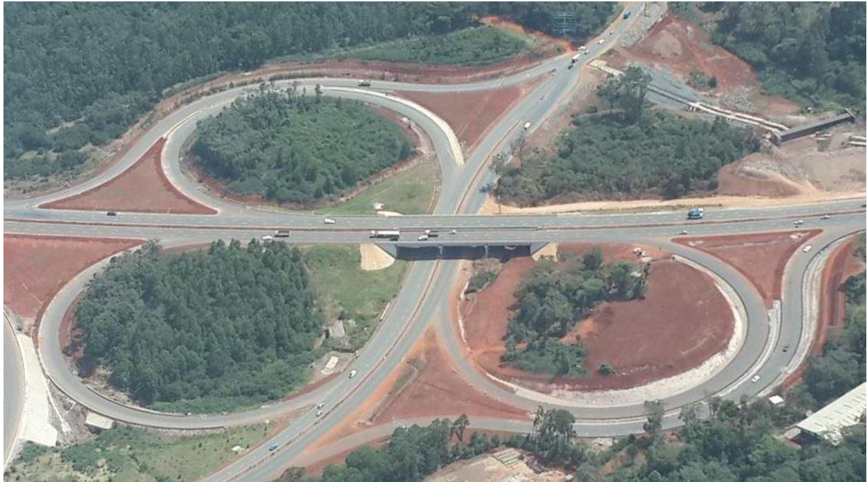
Nairobi South Bypass road in Kenya under construction
